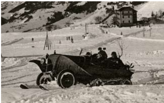
Left: Surely not a standard car! B2 Caddy Sport with track and snow equipment during a test in Haute Savoie, with Lucien Rosengart behind the steering-wheel. This picture is from a postcard - several photos exists from the same occasion.
