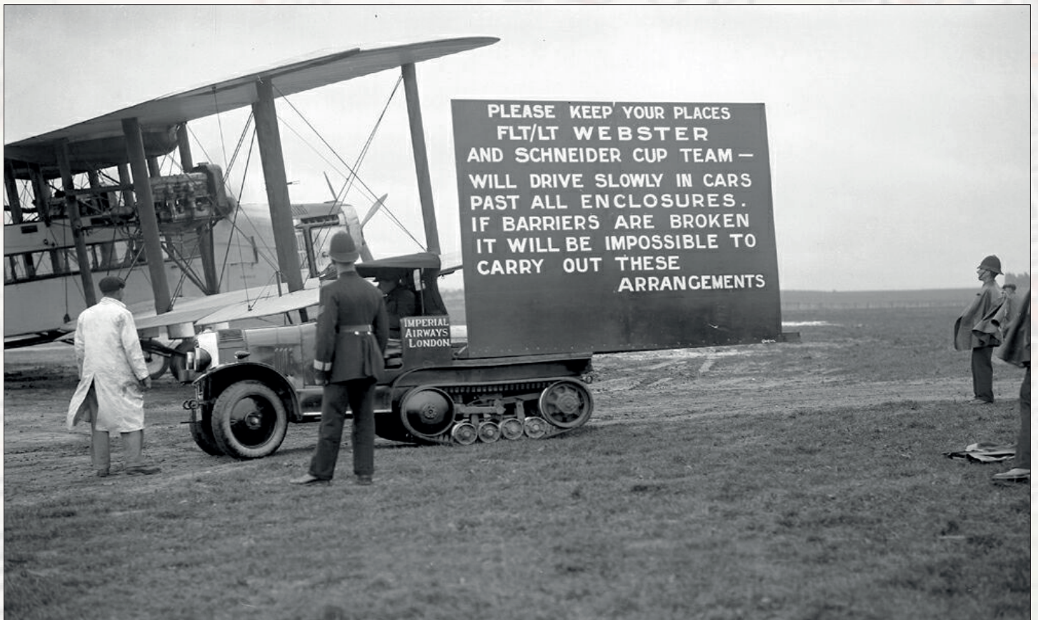
Citroën-Kégresse P4T flat bed. Three engine Handley Page Type W, 25 built, in service from 1921 until 1934
